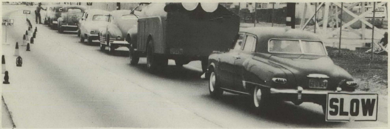
Method for setting up equipment and stopping traffic on four-lane highway.
