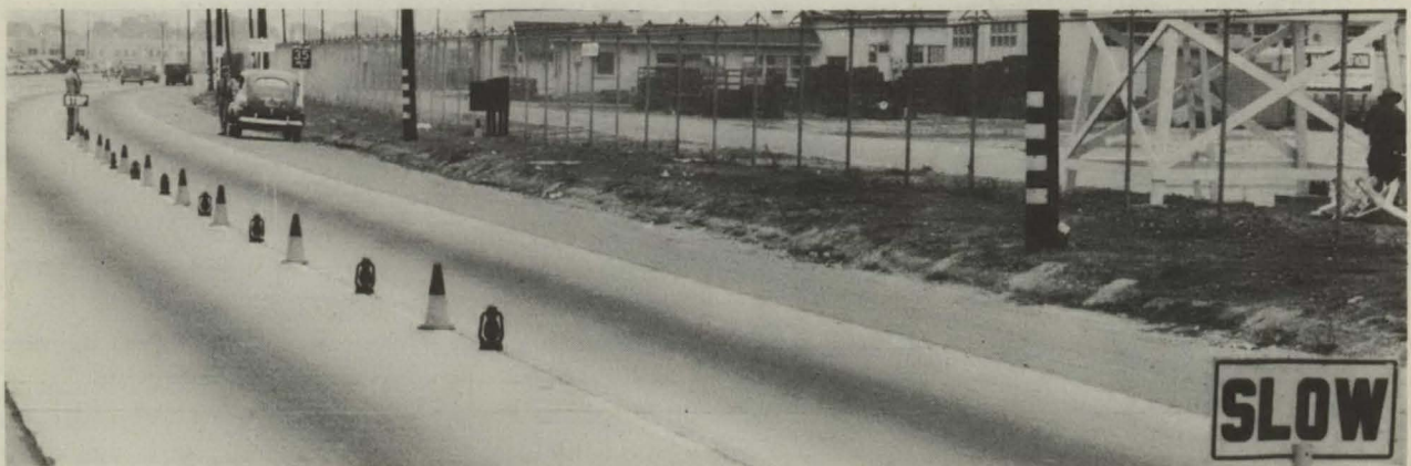
Method used in setting up equipment and stopping traffic on a two lane road.
