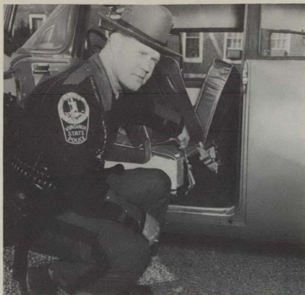
Lt. F. A. Bradley, Jr., holds safety belt strap attached to turnbuckle which is anchored to steel plate beneath the floor.
