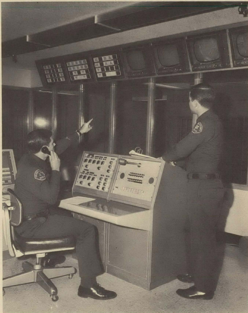
On each floor of the new jails, there is at least one central control room as shown above. Inmates and staff approach security glass in background. At top of photo are panels showing status of every door leading out of the security section plus television monitors for critical areas. Console is for electromechanical control of doors and intercom. At left edge of photo is console for internal phones and audio monitoring devices.
