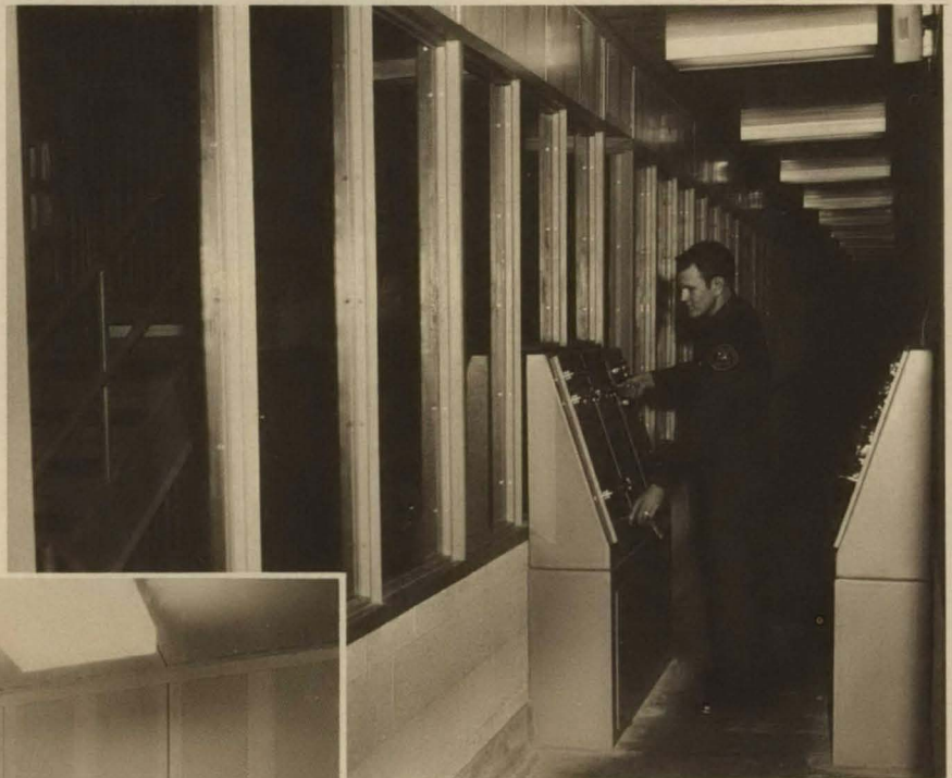
Deputies control individual doors to modules from control panels located in glass-enclosed walkways. The catwalks run between parallel double-tiered cell blocks, and there are no out-of-sight areas in any of the cells.
