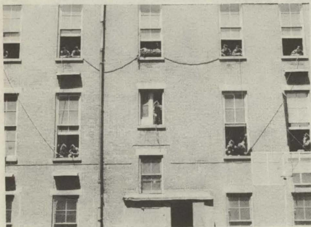
Figure 11.—Net in position to be dropped. Main lines and guy lines in place.
