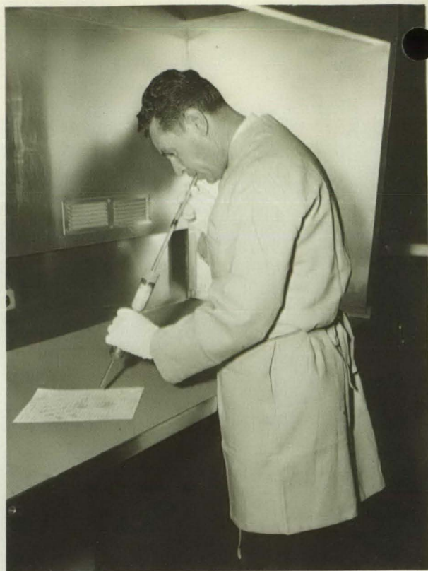
Developing latent fingerprint impressions with an iodine fuming gun.
