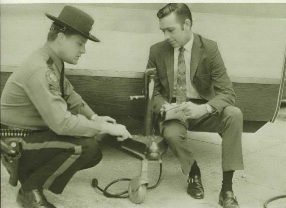
State motor vehicle division inspector and supervisor examine trailer hitch for evidence of tampering or serial number alteration.
