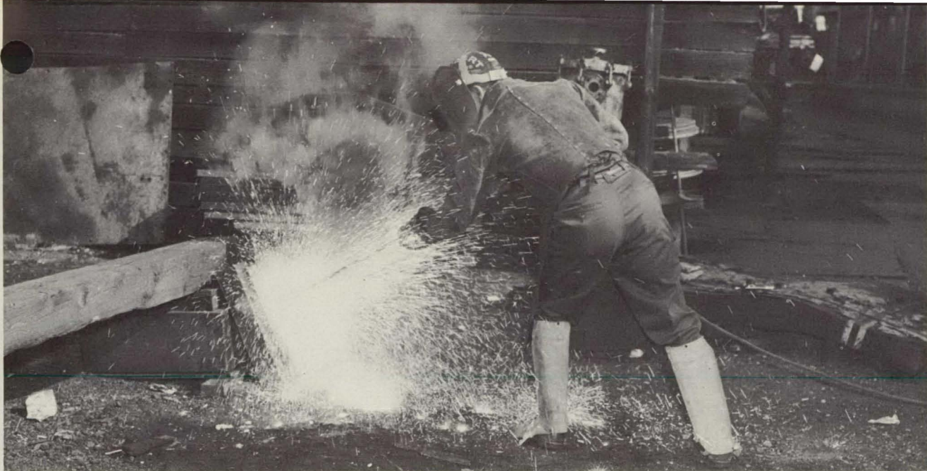
The burning bar consumes itself and gives off a spray of sparks as it penetrates tempered steel.
