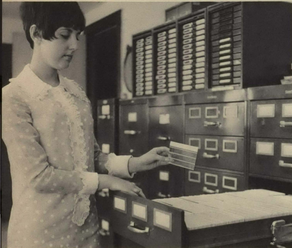
Saved space is a definite advantage in microfilming, for one file drawer now holds 6,000 records.
