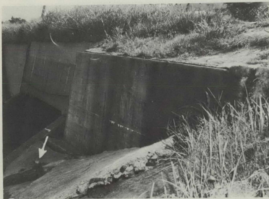
Figure 4.—Concrete embankment with large stump at base.
