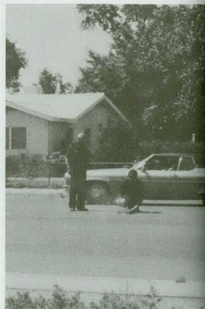
Police car is positioned to protect officers while they paint markers for stopwatch zone.
