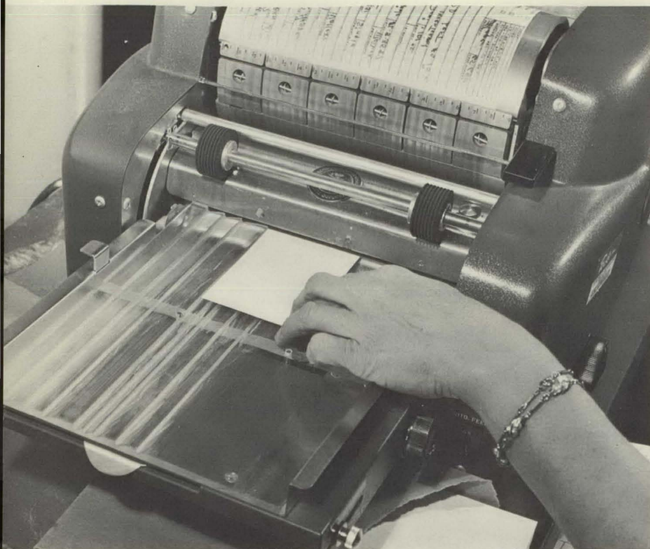
With master copy in place on the fluid duplicator, a 3 by 5 card is run through for indexing of the report.
