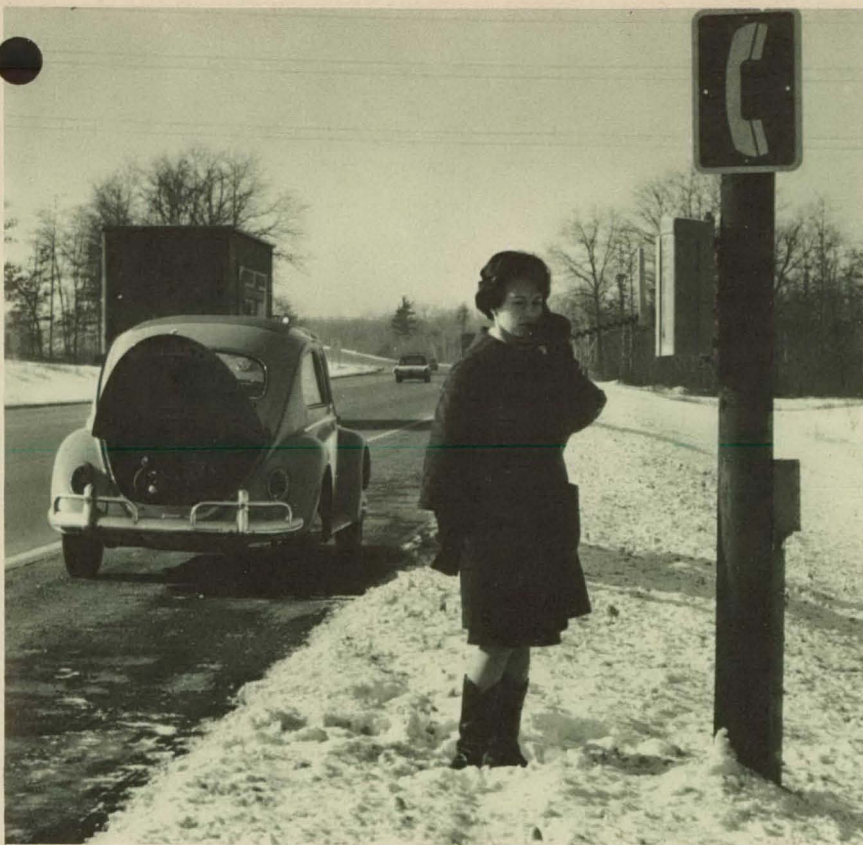
Telephone package is mounted on wooden pole 12 feet from outside edge of driving lane.
