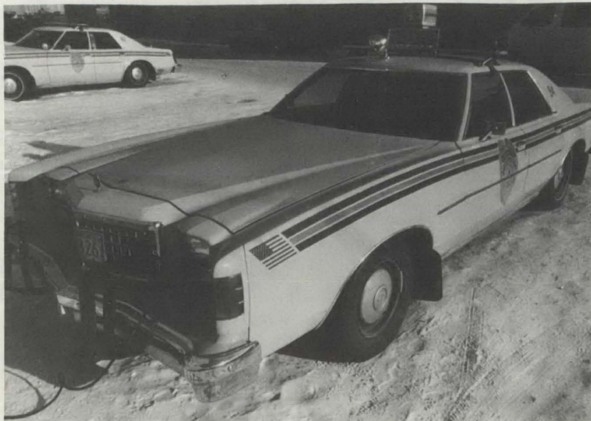
A patrol vehicle "plugged-in" to keep the engine warm. Note the cord extending from the grille area.
