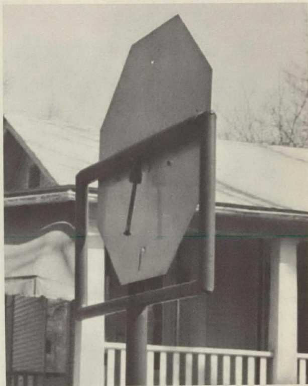
Mechanism showing how sign is attached to upright.
