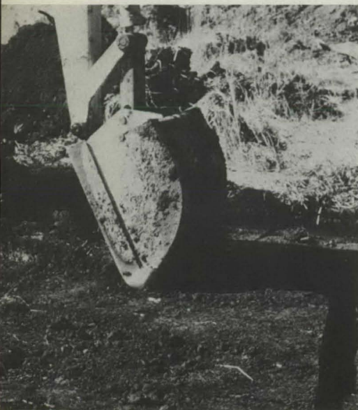
Figure 4. A backhoe with a nontooth bucket leaves a smooth surface.
