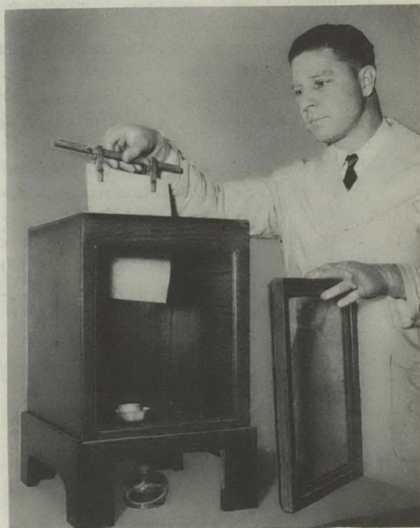
Iodine fuming cabinet in use.
