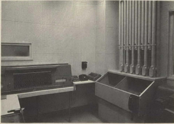
Portion of the Teletype room. On the left is the control console for the police call box system. To the right is the master station for the pneumatic tube system.
