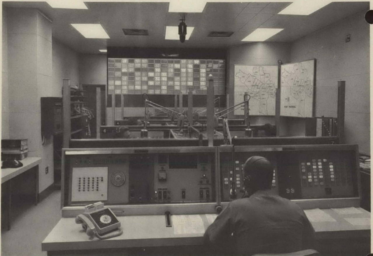
Seven-position communications console for handling all radio and complaint telephone traffic.
