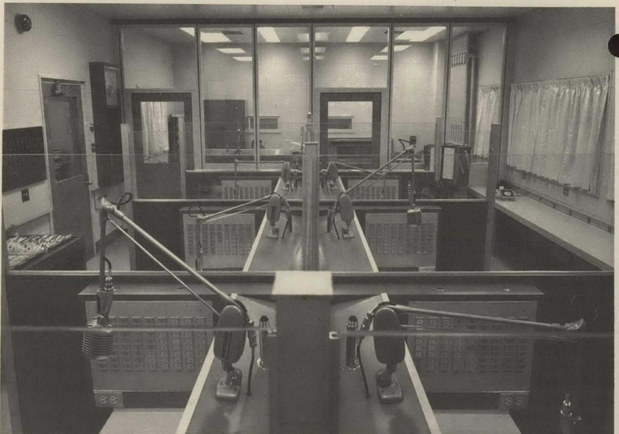
Six communications dispatching positions. To the right is shown a section of the "Disaster Counter." This counter is equipped with ring-down telephones to the emergency services of other municipal agencies.
