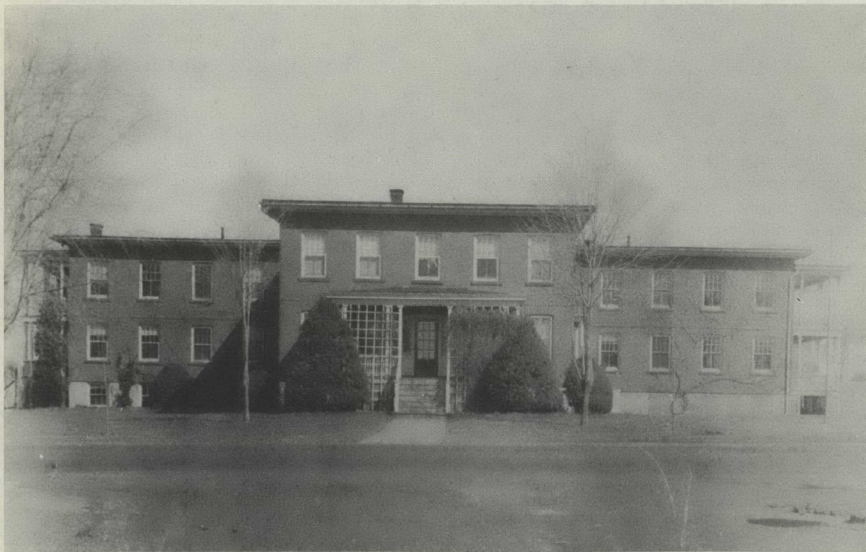
Almshouse before renovation.
