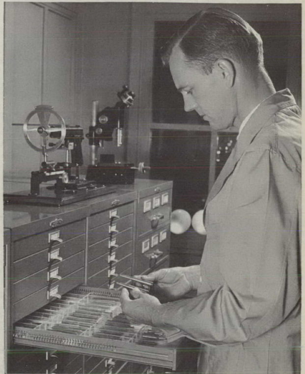
The Standard Ammunition File in the FBI Laboratory permits comparisons of such characteristics as bullet composition, weight, diameter, base and nose shape, and cartridge case markings.
