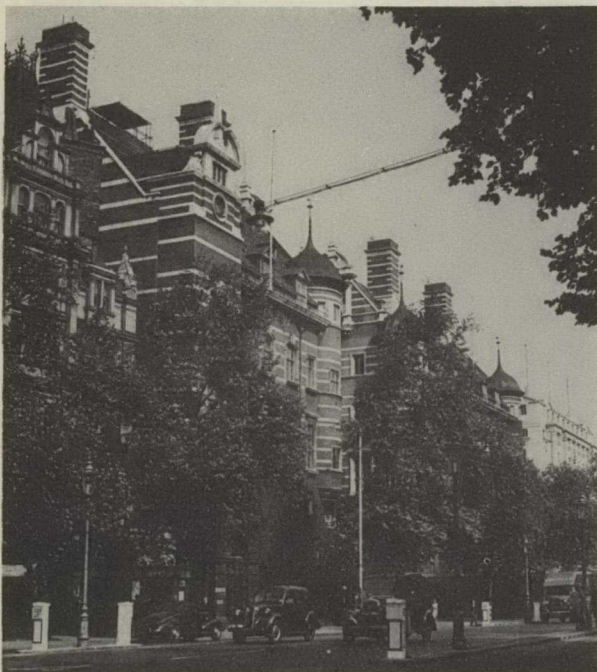
Thames embankment entrance of Metropolitan Police Headquarters.
