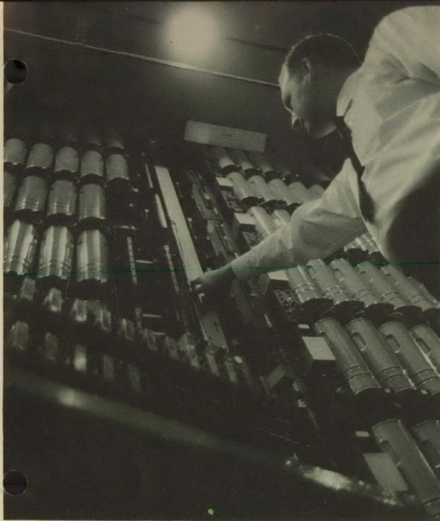
Special line identification equipment enables a telephone company switchman to identify the specific telephone from which an annoyance call was placed.
