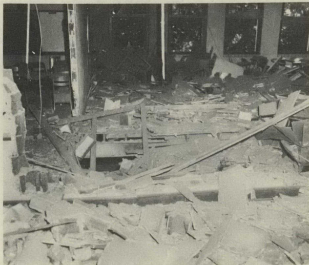
Bomb damage to a school.
