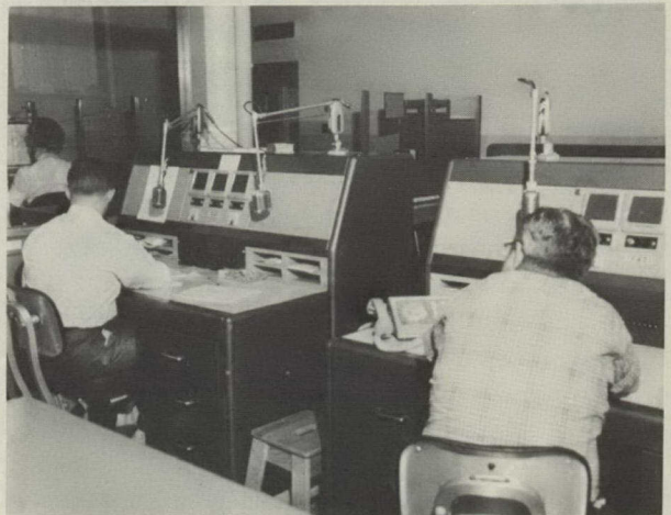
Dispatching consoles for police radio communications.
