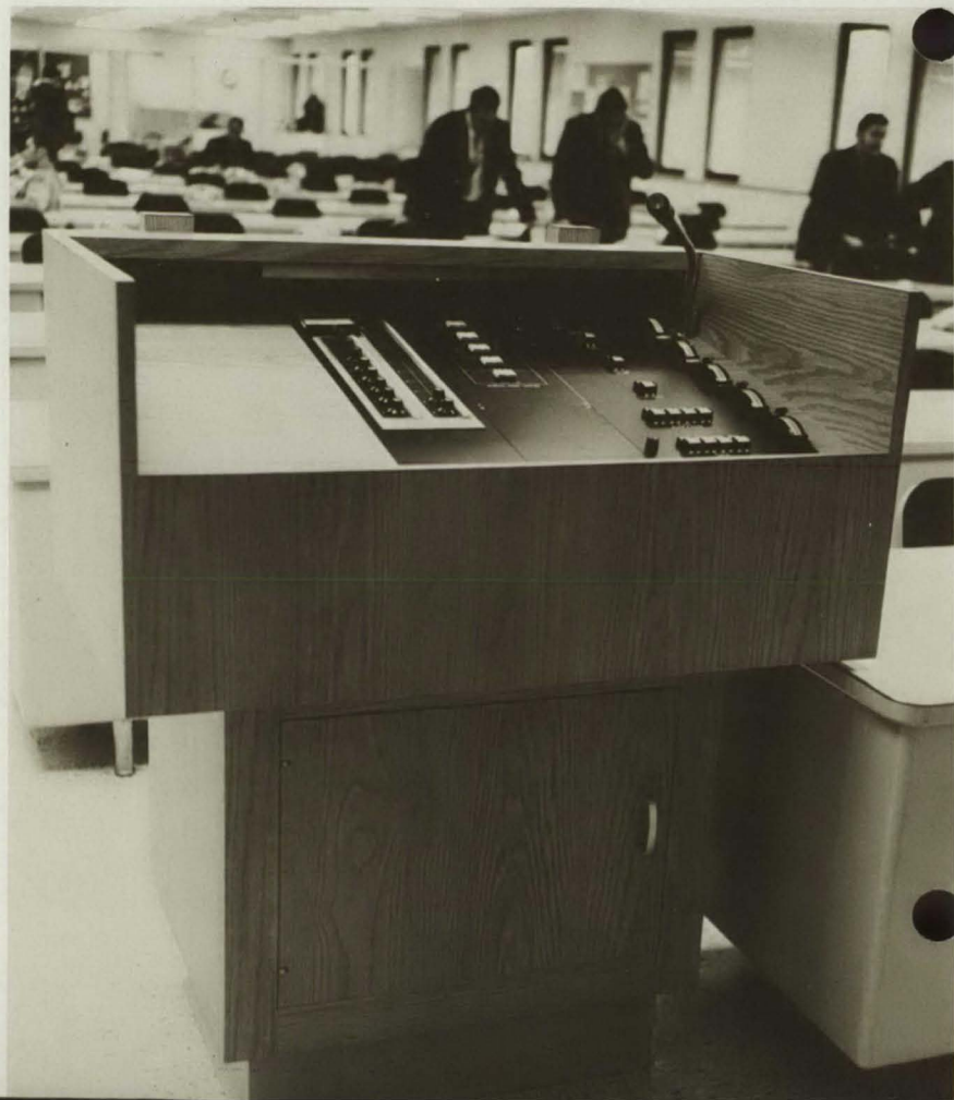
From this rostrum in the detective bureau assembly room, an officer can control lighting effects and projection of crime scenes on a screen.
