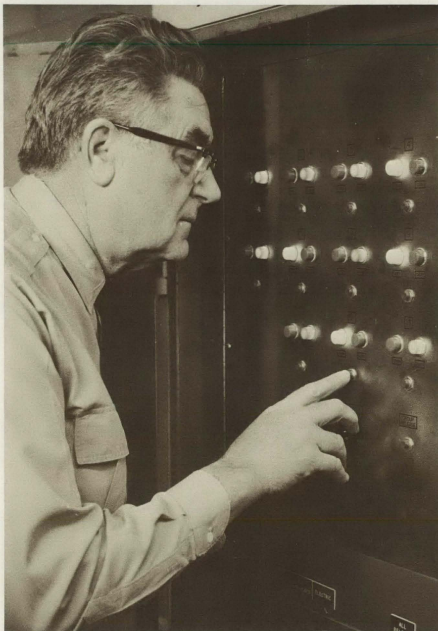
Pushing a control panel button, an officer may lock or unlock individual or a group of cells by electrical or mechanical means.
