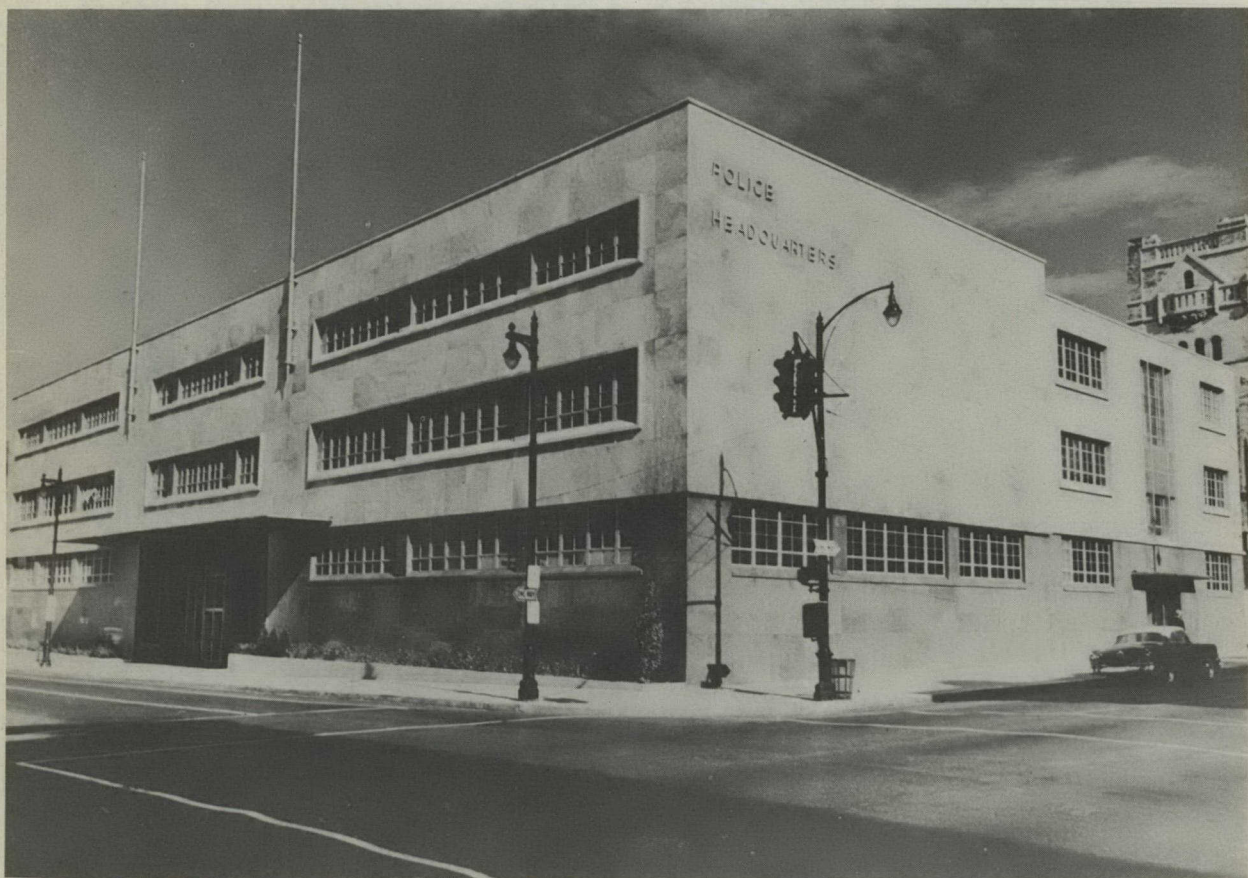
Louisville police headquarters building with lower portion in Texas red granite and upper part in Vermont green-gray marble.
