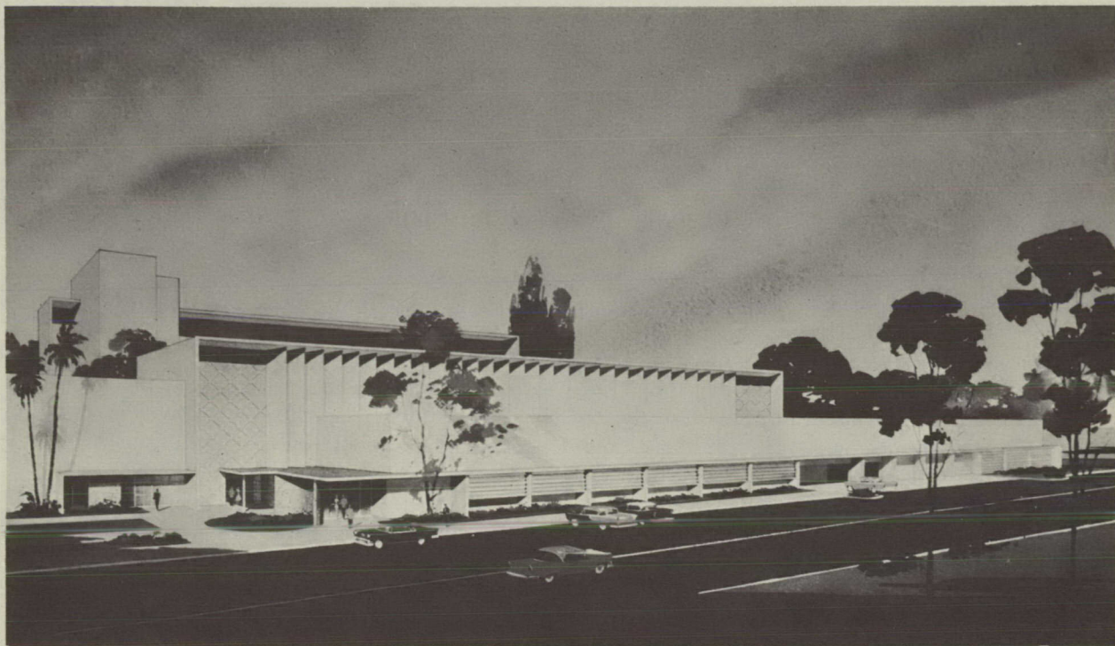
Kern County Sheriff's Department Facility, Bakersfield, Calif.
