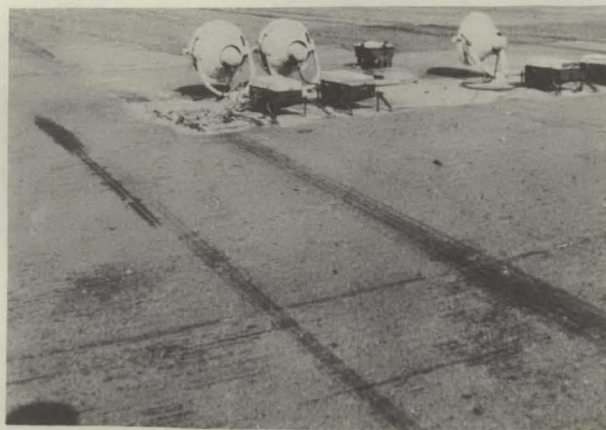
Nest of landing lights struck by plane.
