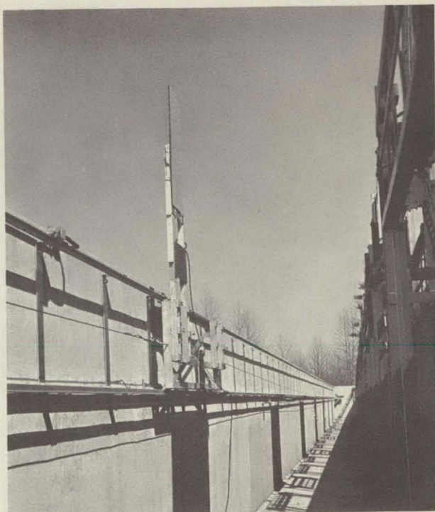
The 190-foot track, shown here with target mounted, extends the length of the rifle range butts. The target travels the distance in 16 seconds.
